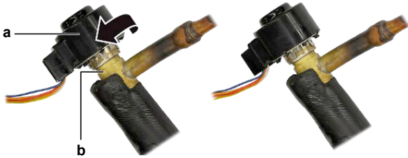
a Expansion valve coil b Pipe
